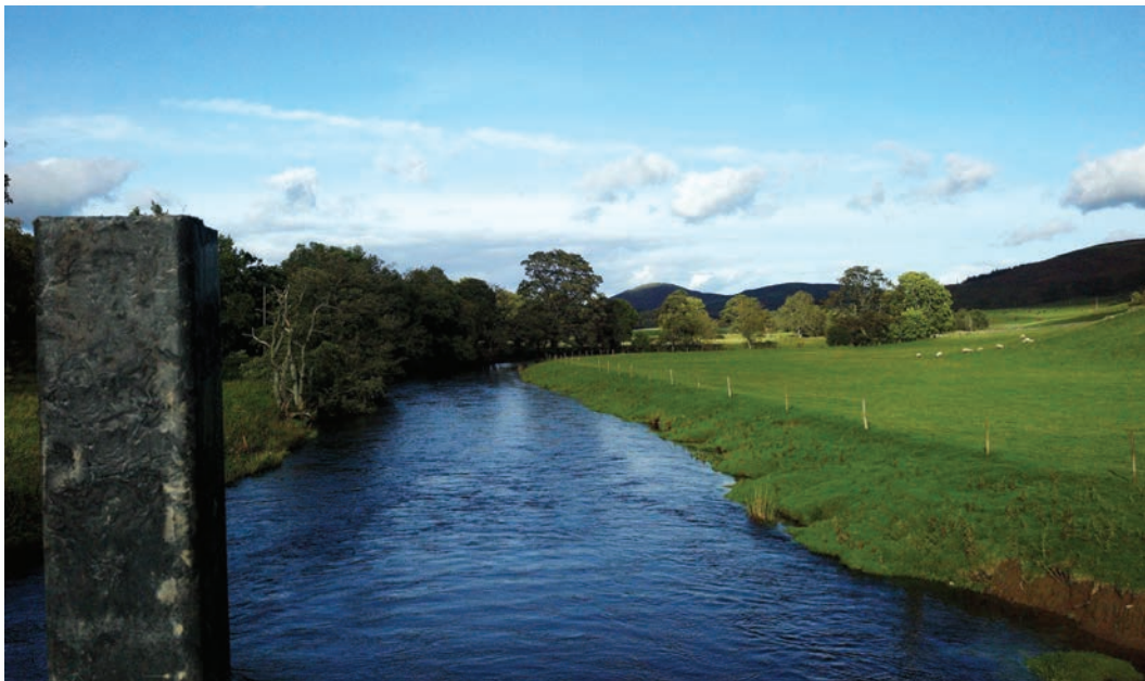
Above: The site of a 'heavy-goods' vehicular bridge built using our STRUXURE® Pre-Built Bridge Panels in Peebleshire, Scotland. Opposite: Various installed ECOTRAX® Composite Railroad Ties and STRUXURE® Composite Infrastructure Products.
