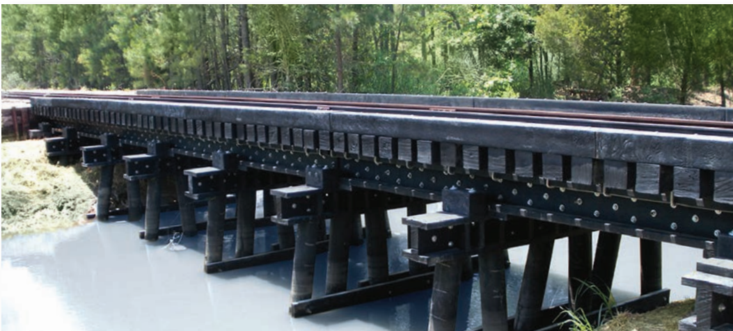
Top: A heavy-load bridge built with STRUXURE® Composite Infrastructure Products at Fort Bragg, NC. Above: A railroad bridge built with ECOTRAX® and STRUXURE® Composite Infrastructure Products in Fort Eustis, VA.
