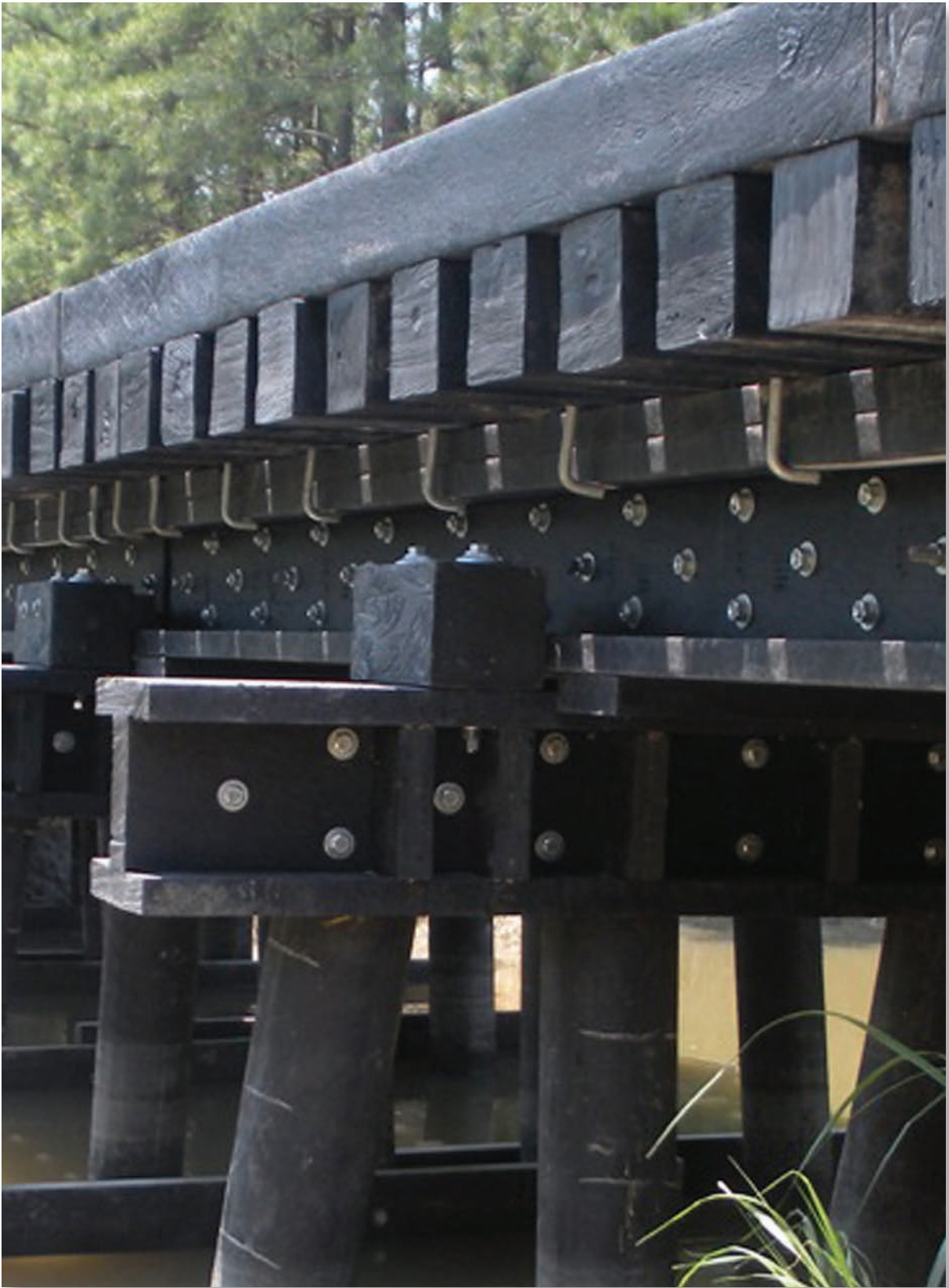
Above: Railroad bridge built with ECOTRAX® Composite Railroad Ties and STRUXURE® Composite Infrastructure Products in Fort Eustis, VA. Opposite: Installed ECOTRAX® Composite Railroad Ties on a transit line near Dallas, Texas.
